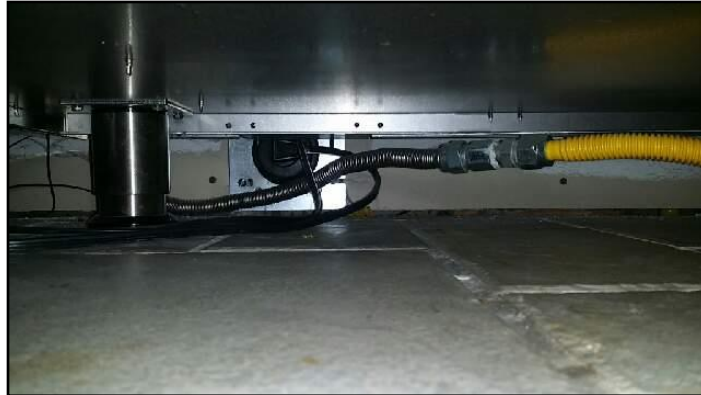
Missing shut off valve
