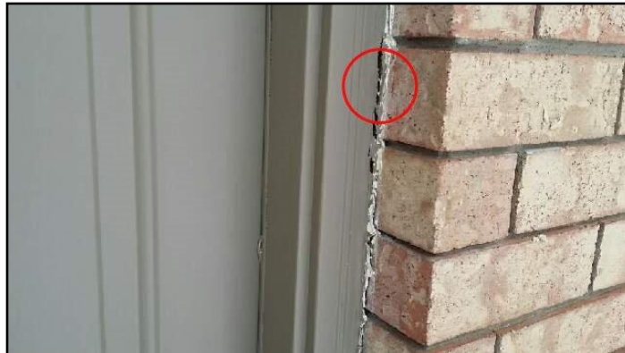
Caulking missing or ineffective
