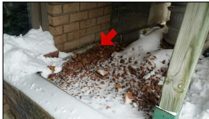
Improper slope
