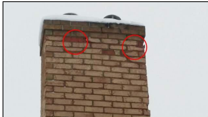
Loose, missing or deteriorated masonry
