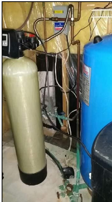
Oxidized supply lines
