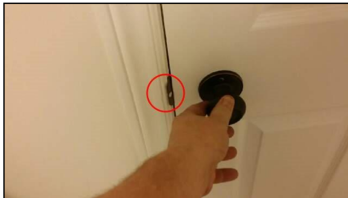
Does not latch properly
