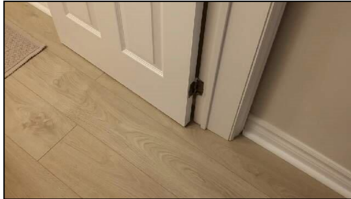
Loose or poor fit
