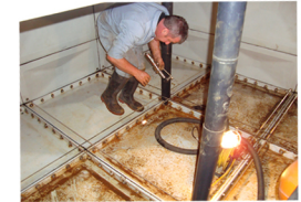
Tank refurbishments & repairs
