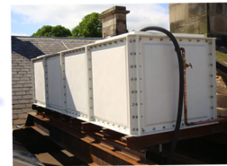
New installation of GRP tanks
